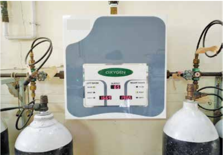
A Large Public Sector Hospital Karachi
